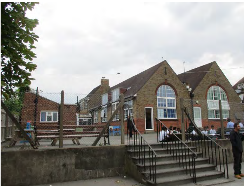
Rear of original building
