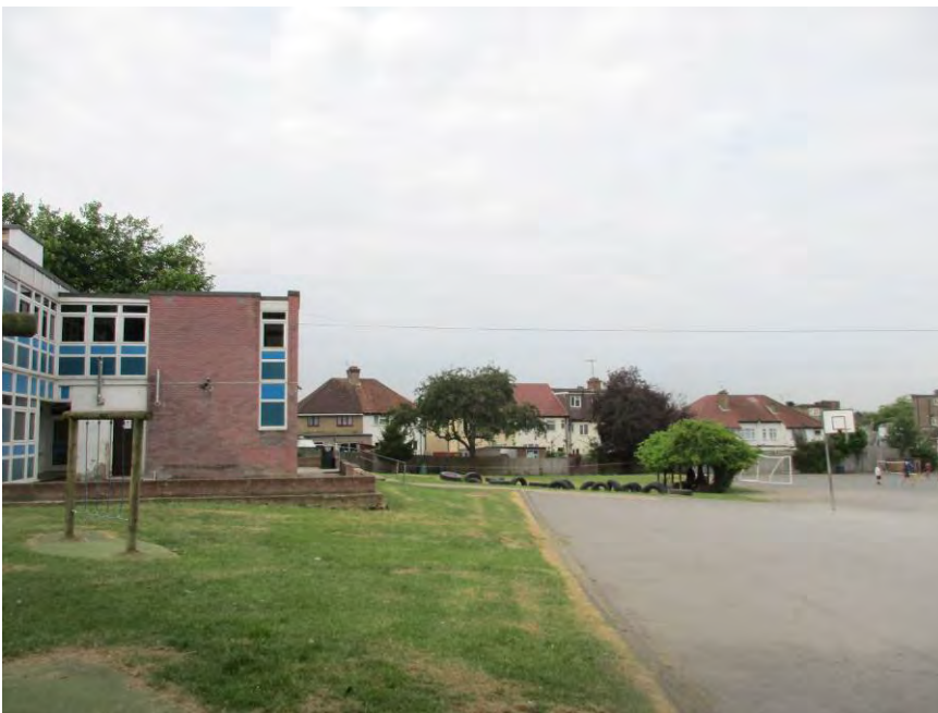
Looking towards existing kitchen building and houses on Roxeth Grove
